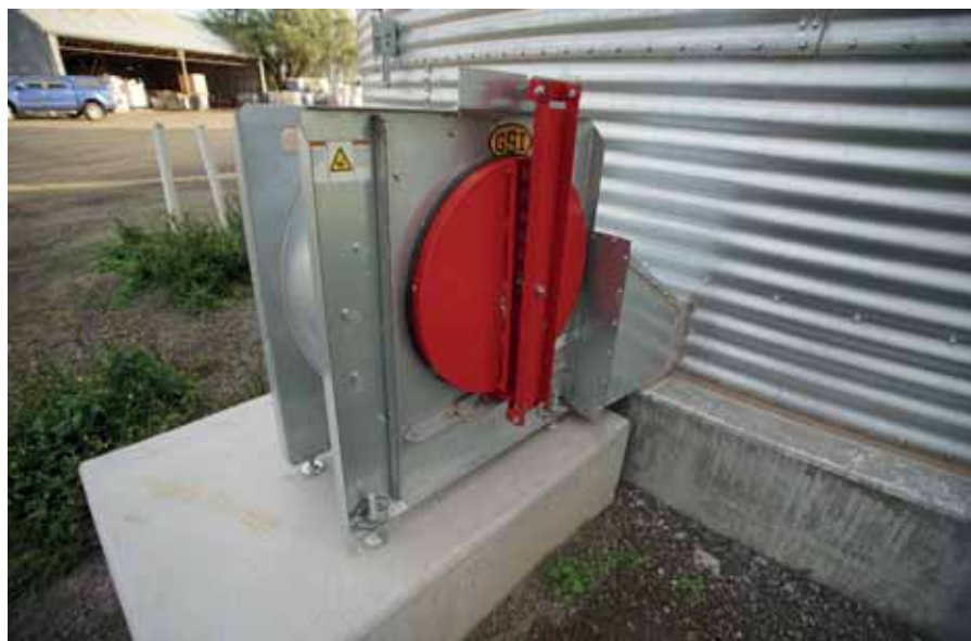
Aeration: GSI badged aeration fans curiously feature a seal plate, but the silos do not meet AS2628 for fumigation.
