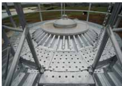
Top lid: Sturdy access steps and railing surround the inlet lid
