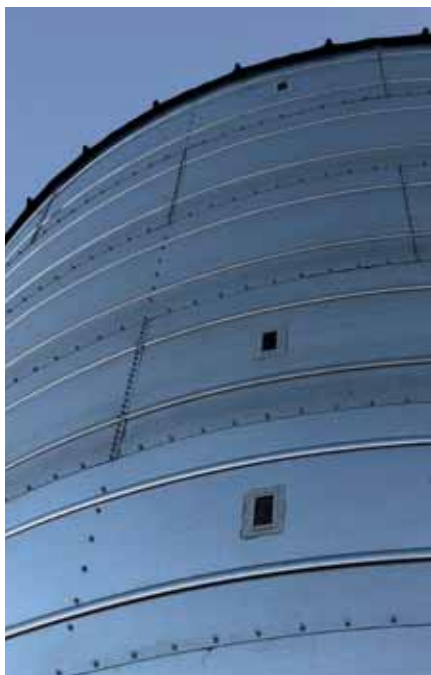
Walls: Wall thickness and galvanising grades can vary between silo manufacturers, makes and models.
