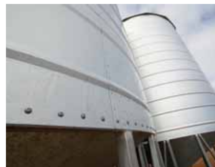
Wall: Wall joins are overlapped and solid riveted with two convex ribs per wall section ring.
