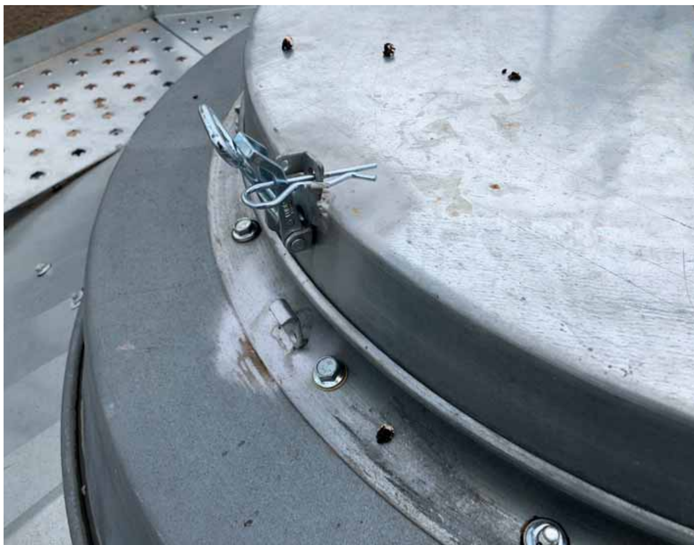
Over-centre latches are prominently used. But make sure they won’t accidentally latch when you don’t want them to using an R-clip to secure them in the open position.
