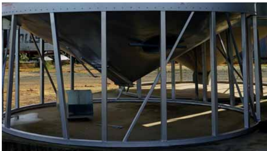
Base: Fabricated using SHS with vertical and angled uprights to accommodate larger auger hoppers.
