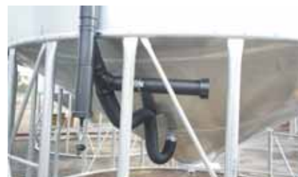
Neatly butt-welded HDPE plumbing on the HE elevated cone base gas-tight sealable silos.
