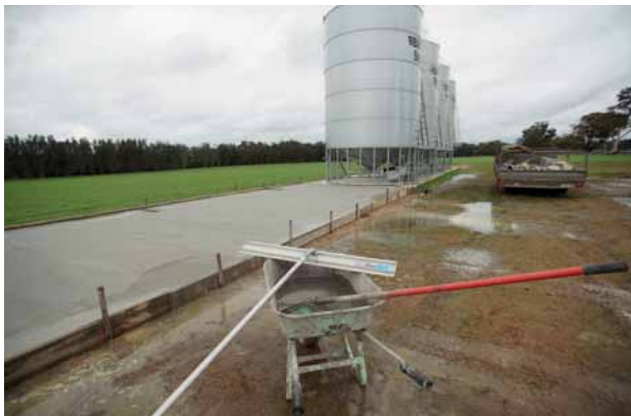
Laid: Foundations may need to be built to prescription depending on the silo and the soil type.
