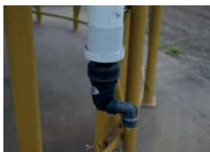
Drainage: A self-emptying water trap fitting built into the thermosiphon.
