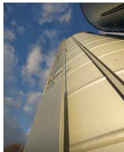
Cageless: A relatively narrow ladder and lack of cage or roof-top rails needs to be rectified.
