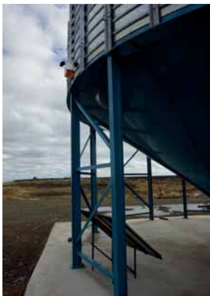
High valve: At over three metres off the ground, the valve is too high to service or read for pressure testing without a step-ladder.
