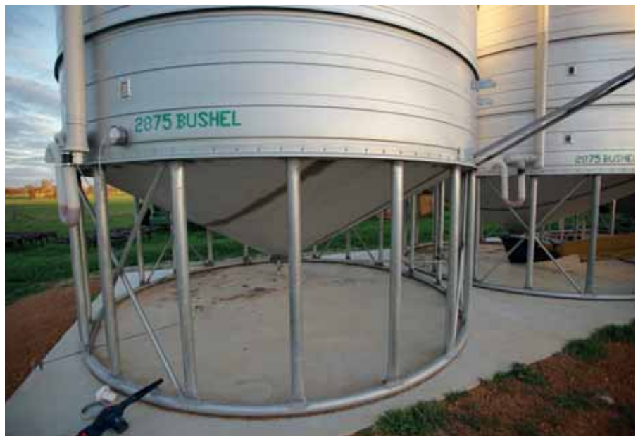
Galvanised: Duragal SHS and RHS does not carry as much galvanising as the hot dipped steel in these examples, with the latter also benefiting from internal galvanising protection.
