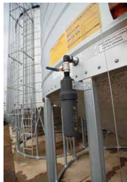
Phosphine application: Poorly designed, the canister does not allow phosphine tablets to liberate, potentially under-dosing insects and creating resistance.
