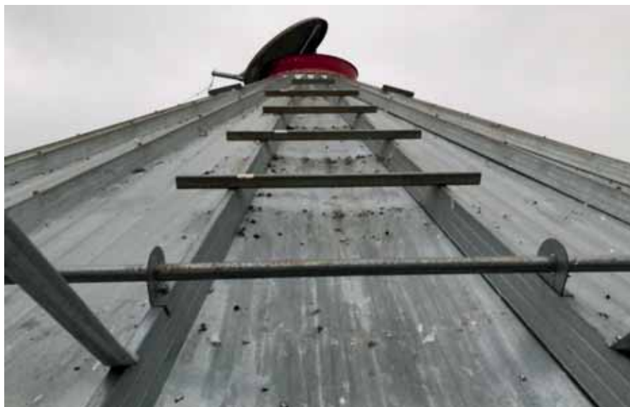
Rooftop: A ground operated lid means that these basic rooftop rungs should rarely be required.
