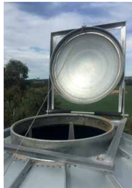
Inlet lid: The release cable remains in the centre of the lid in the fully open position providing an obstruction when filling.
