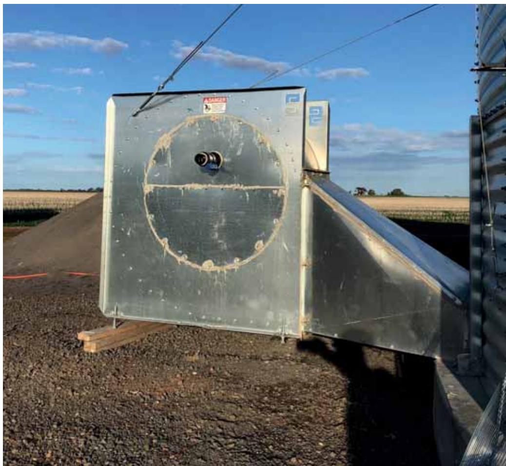
Seal plate: Large capacity fans pump air through a full floor for drying but sealing these requires a more permanent solution than removal of the grille and attachment of a sealing plate with bolts and polyurethane sealant.
