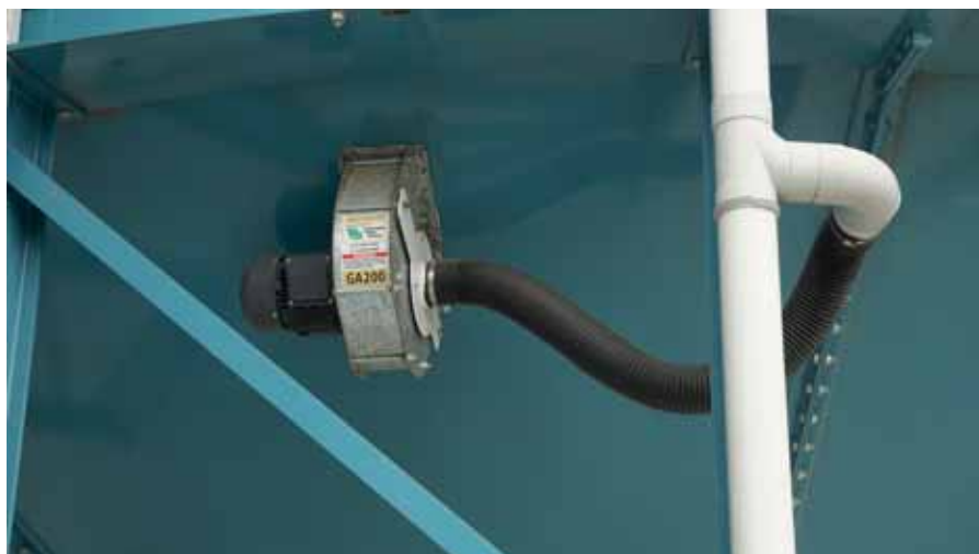
Recirculation: One of the two aeration fans on this 450t elevated cone base is plumbed into the thermosiphon from the headspace.
