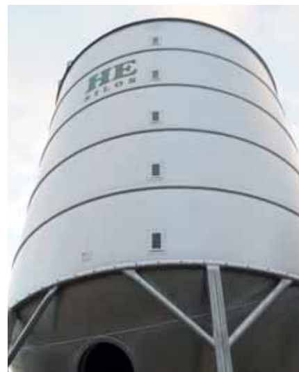
Windows: Each wall section has a top and bottom convex rib and a window at the base to monitor grain level.
