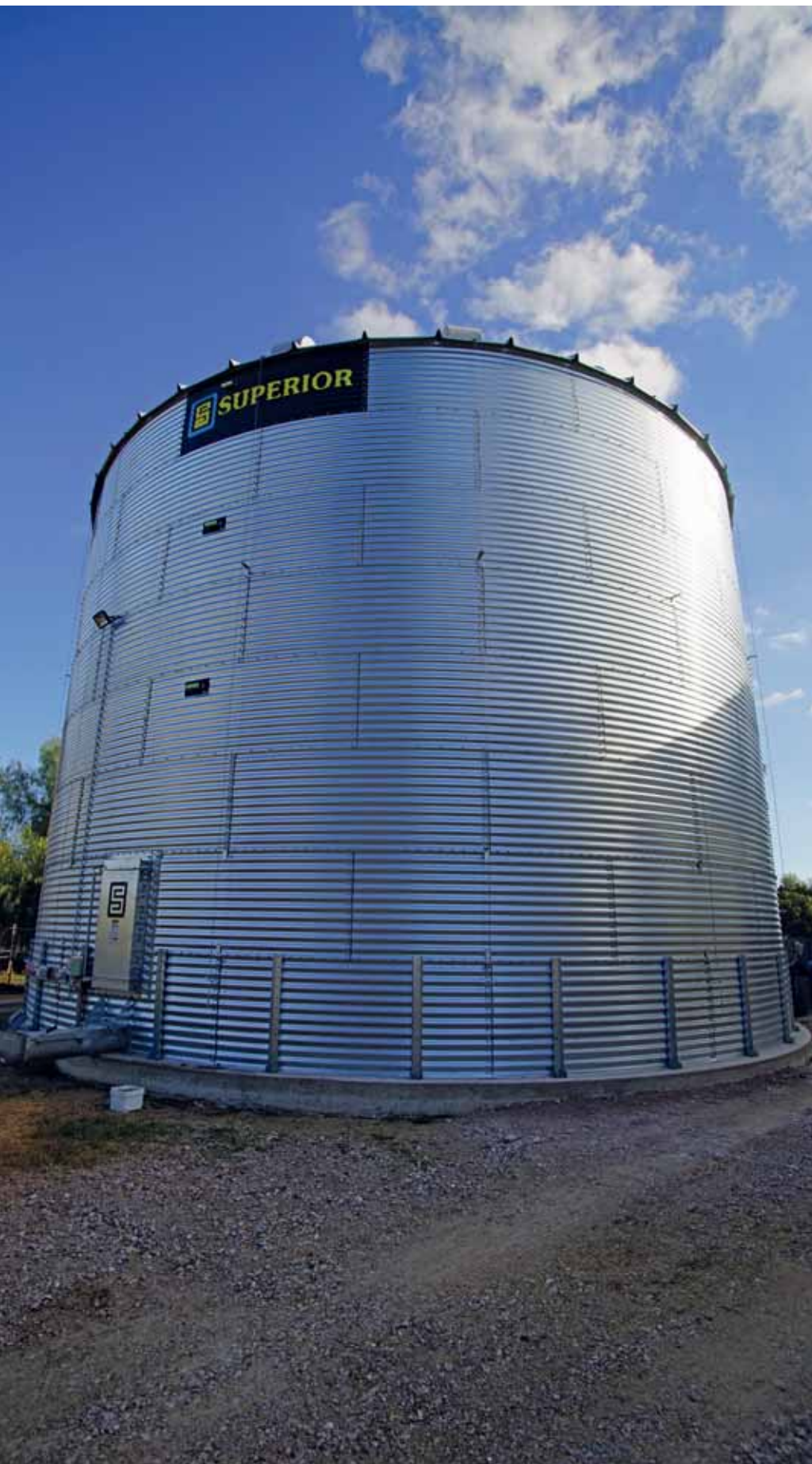
Access: Revised since we inspected them in 2015, the steps to the top now include a mid-way and top platform.
