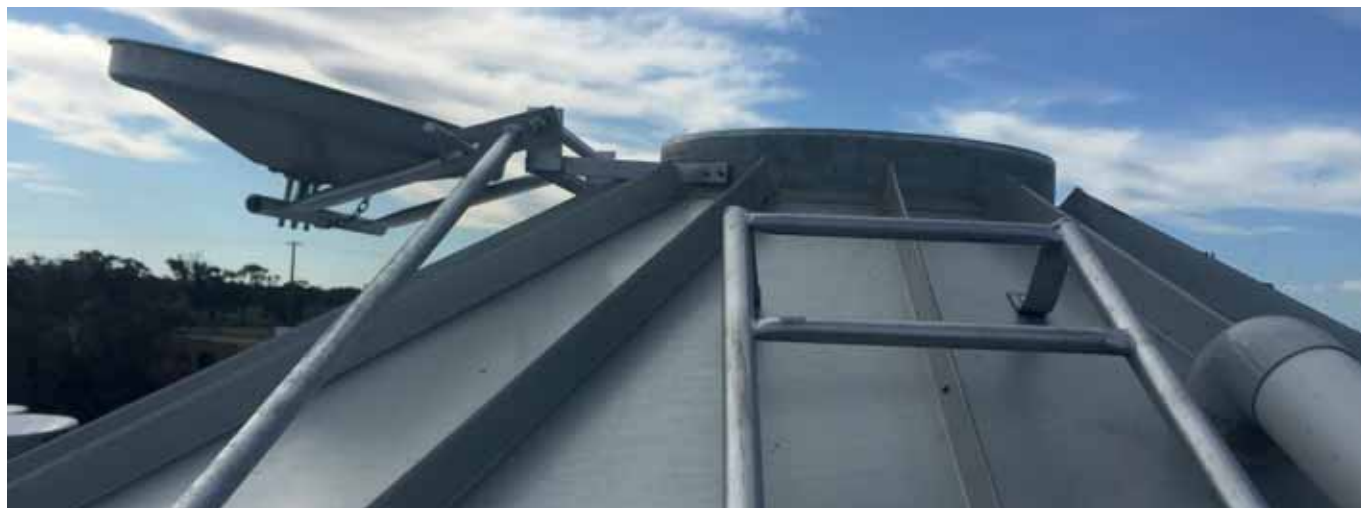
Top lid: The flip-over lid is ground operated and pressure applied with a spring to the centre to provide a uniform seal.
