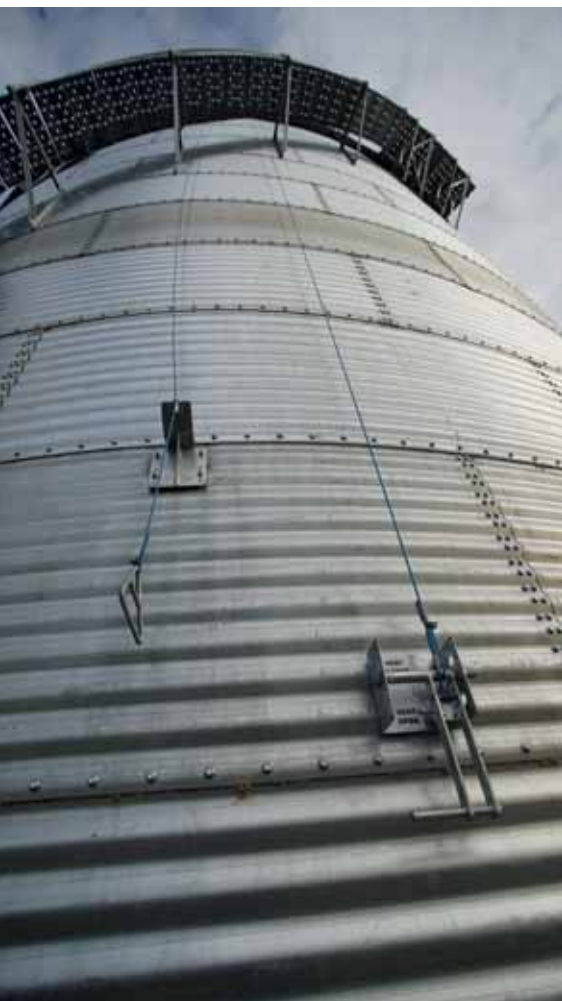
Remote control: Ground operated lid and aeration exhaust vents are operated by wire rope.
