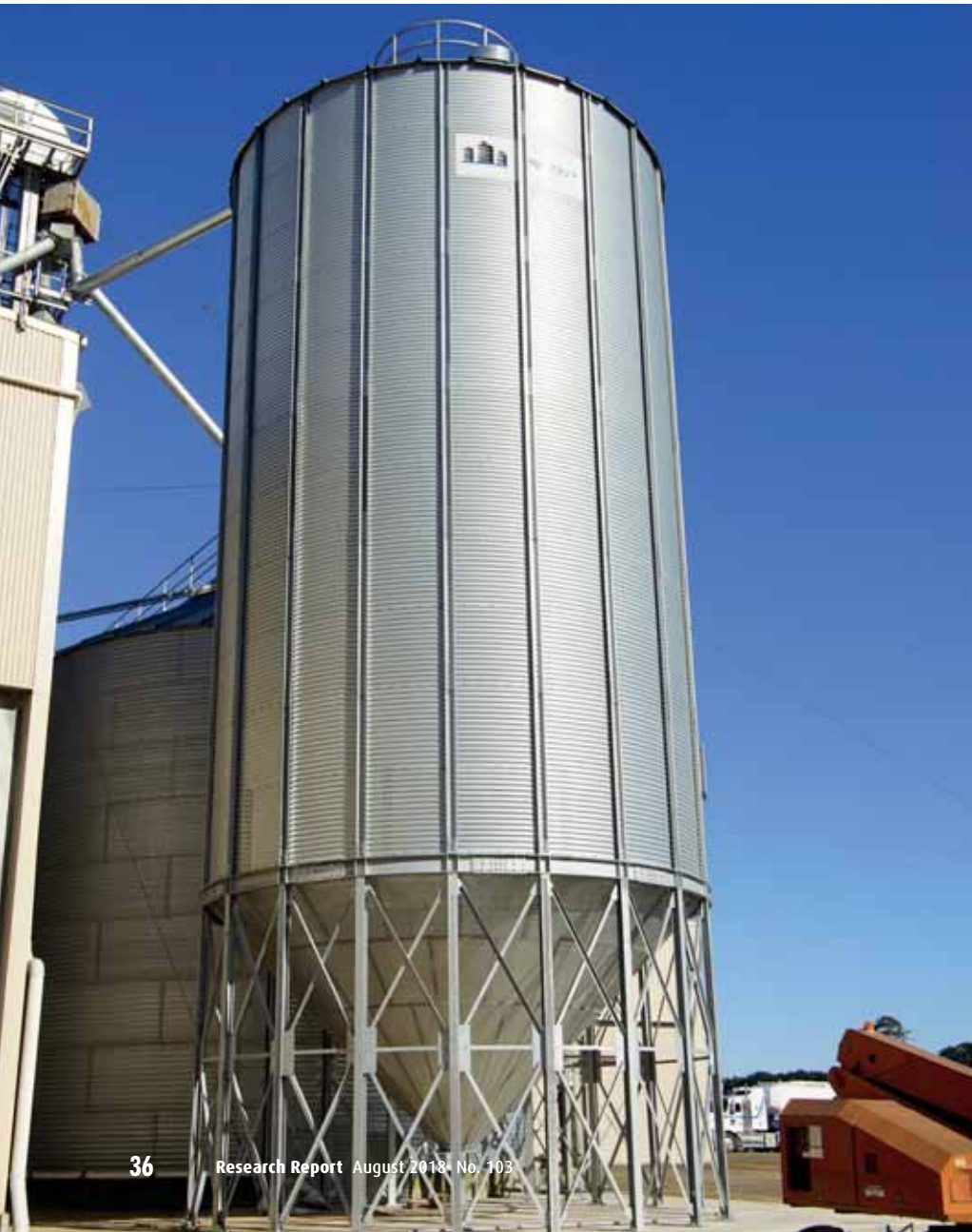
Platform: Crows-nest has a solid platform and railing.
