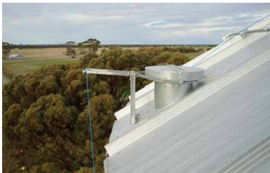
Aeration exhaust: Rooftop aeration vents are well made.
