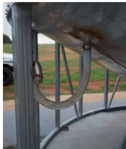
Pressure relief valve: A small cross sectional area and minimal oil capacity of pipe-style pressure relief valves can see them lose oil with diurnal variation.
