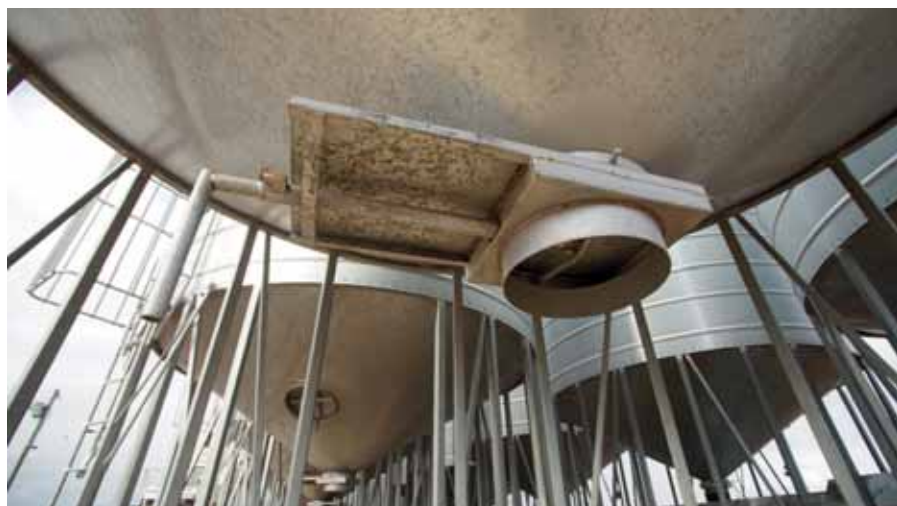
Outlet: The slide gate outlet works well with the ¼ turn sealing mechanism doing the job to assist in maintaining AS2628.
