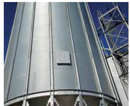
Walls: Corrugated bolted wall sections with stiffening ribs run the height of the silo.
