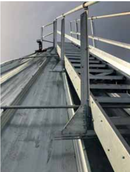
Roof-top: Walkways and handrails on the roof were sturdy on models optioned with roof-top step set and crows-nest inlet platform.
