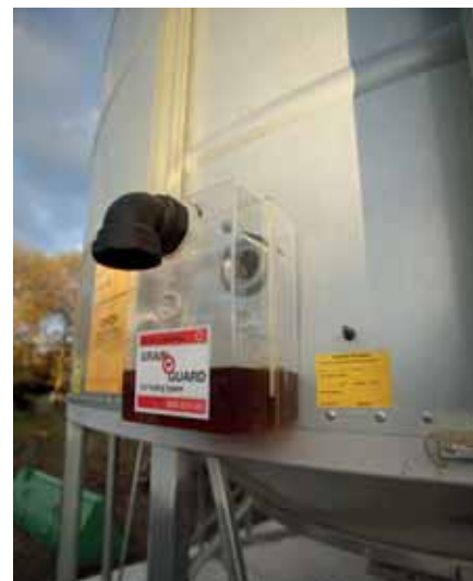
Pressure relief: A GrainGuard valve at ground level with test valve and instructions is easy to get to.
