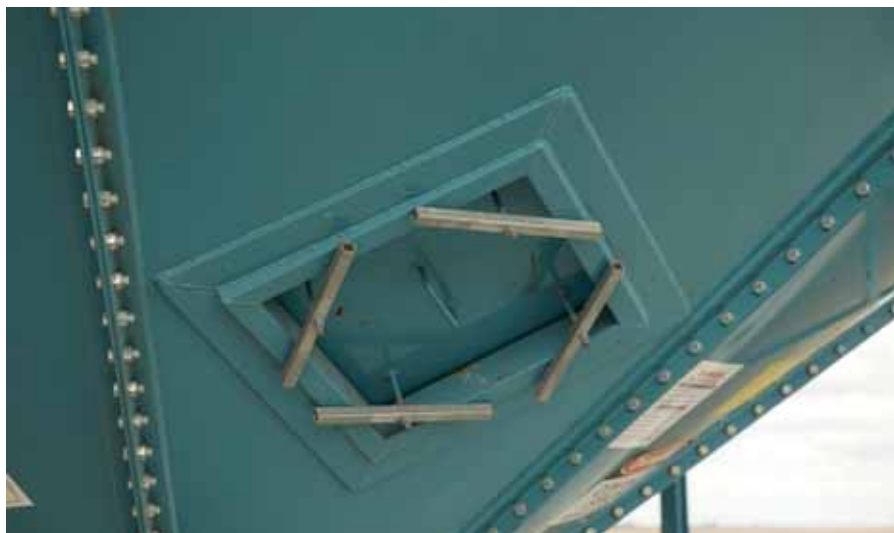
Access: The access door like the rest of the Dennys silo elevated cone base, is solid, but requires tools to pull tight for seal testing when empty.
