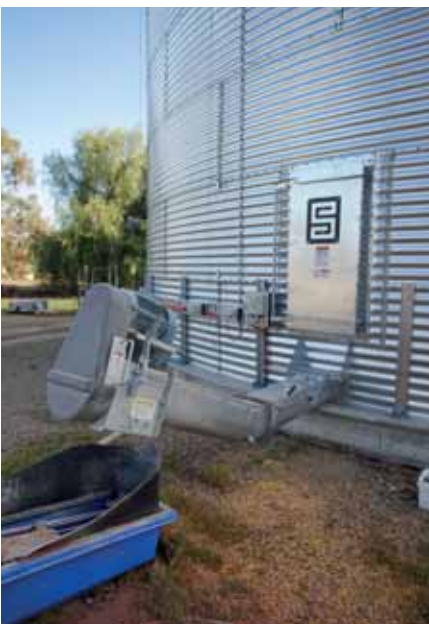
Outload: Springland sweep and outload augers are used.
